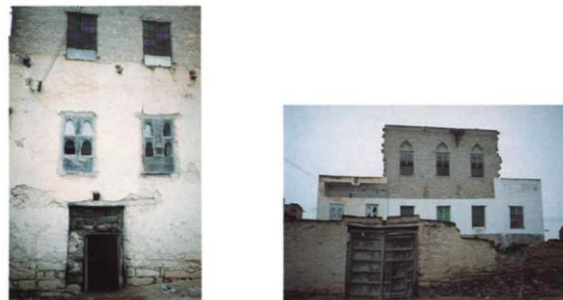
Fig. 13: Big open space in front of house in Salalah (Al-Hinai et al., 1993).
