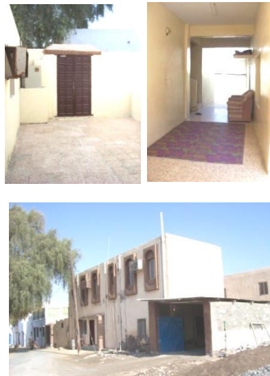
Fig. 11: Front courtyard and cross corridor (source: author)
